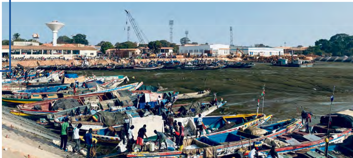
Fig. 1: Porto do Alto Bandim, the main fishing port in Bissau currently under renovation with the support of Chinese foreign aid (Photo by the author, 2022).
