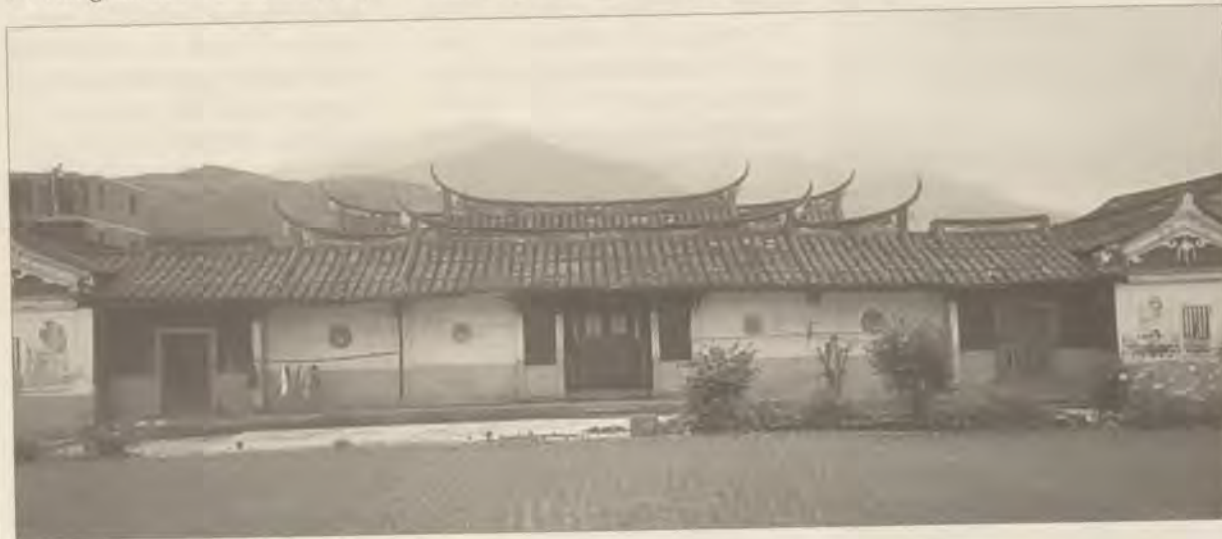
A mansion in South Fujian, China, built in the early twentieth century by a Chinese lineage in Malaysia. It was intended to be used by the emigrants upon their return to China, but that return never happened.
