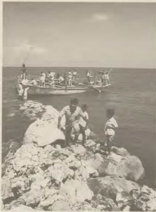
Repairing groyne at KUDEHI ATIRI
