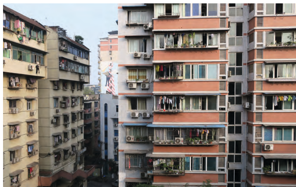
Characteristic apartment houses in Chongqing. Note the self-installed split-unit air-conditioners and the clothes hanging outside due to the high humidity indoors. (Kobi 2017)
