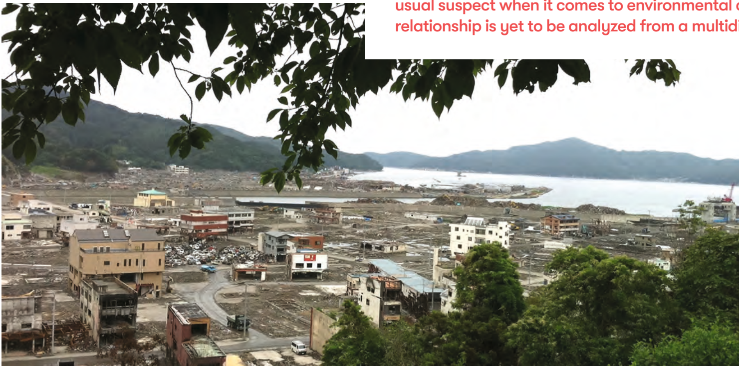
Fig. 1: Earthquake-stricken coast in Otsuchi Town, Iwate Prefecture, Japan (Photo taken by the author, 25 June 2011).
