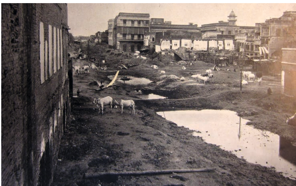
Above: 'Jagannath Ghat Road Construction' (Annual Report of CIT, 1929). Courtesy: British Library.
