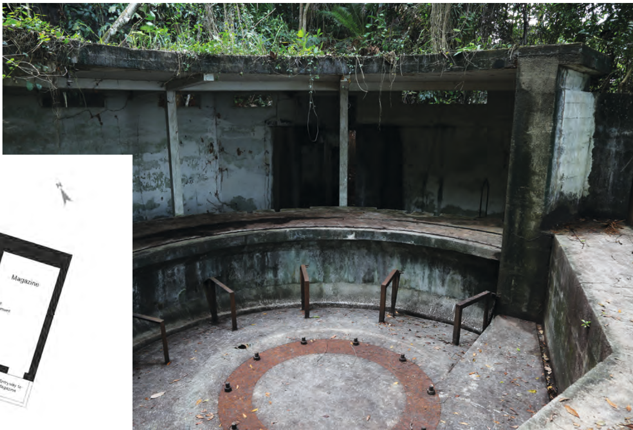
Fig. 2: Gun floor consisting of overhead concrete canopy, gunner's platform, and holdfast bolts for a twin 6-pounder gun. (Credit: Young Wei Ping)
