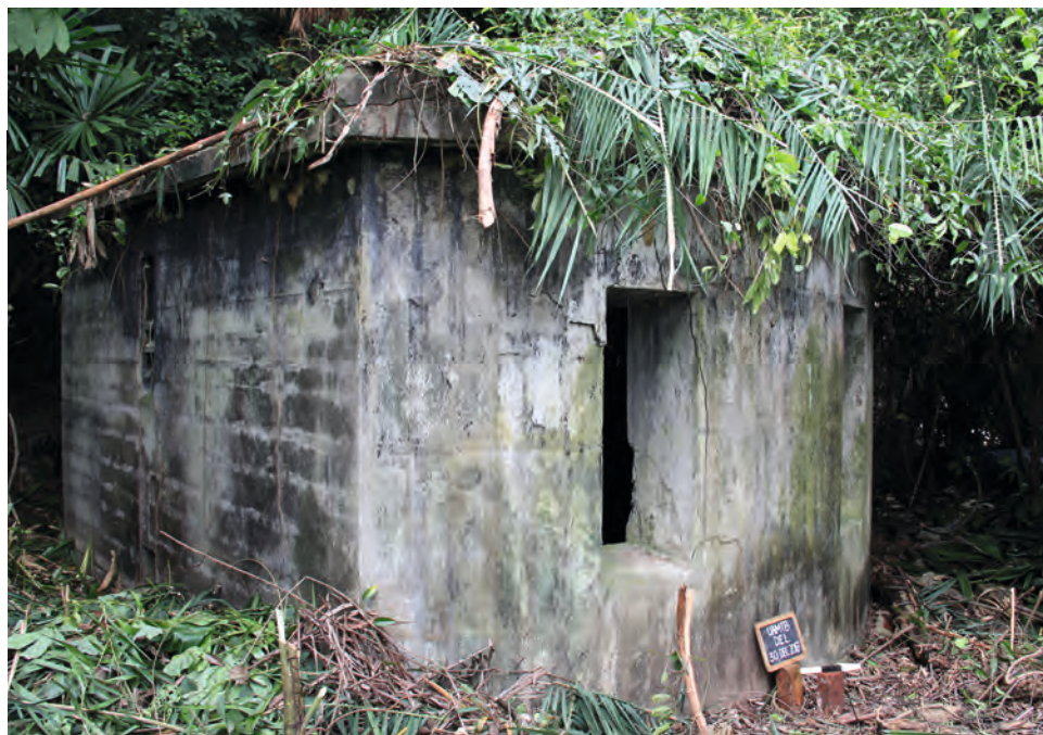
Fig. 3: One of the DEL emplacements featuring steel reinforced shuttered concrete construction to protect the searchlight equipment and crew. (Credit: Aaron Kao)
