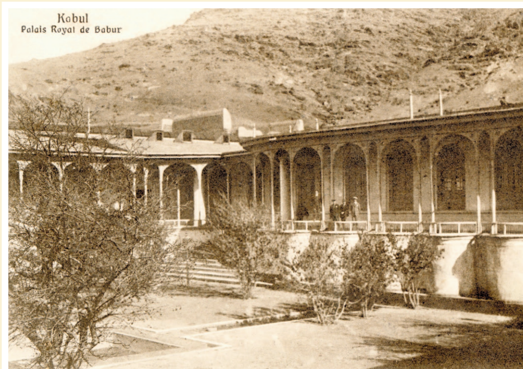
Queen's Palace in Bagh-e Babur, Kabul. 3a (above): In the 1920s (GV 64). 3b (middle): After destruction, 2002 (PB 2002-631). 3c (below): After reconstruction, 2008 (PB 2008-10).
