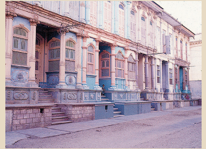
1: Evidence of European influence on traditional dwellings of the Bonra community in Gujarat.
