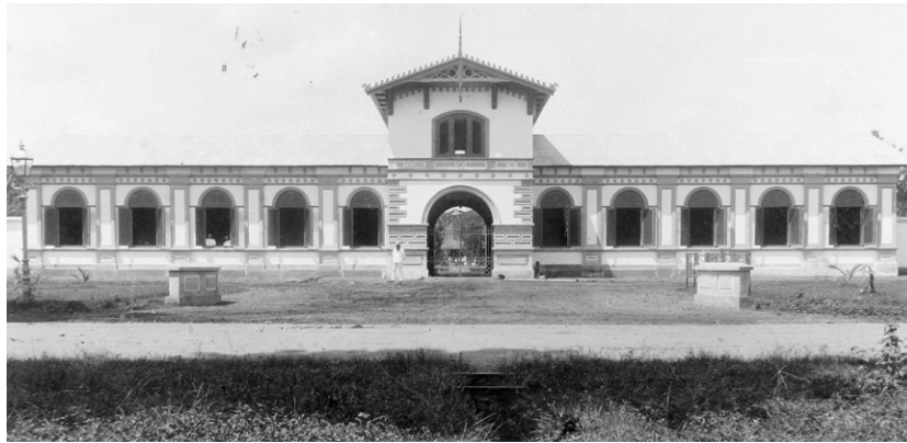
Administrative offices of the opium factory, Weltevreden, Batavia, 1899. The building which housed the Opium Regie appears solid, respectable, and permanent, and gives the impression that Dutch rule can transform even opium consumption into a tool for modernization.
