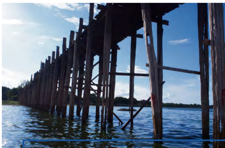
Left: The teak pillars of U-Pein Bridge along Taungthaman Lake in Myanmar. (Photo courtesy of Zin Mar Latt)
