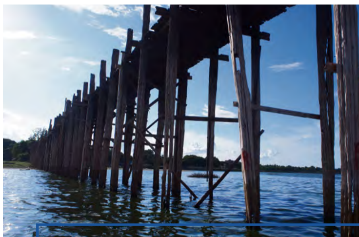
Left: The teak pillars of U-Pein Bridge along Taungthaman Lake in Myanmar. (Photo courtesy of Zin Mar Latt)
