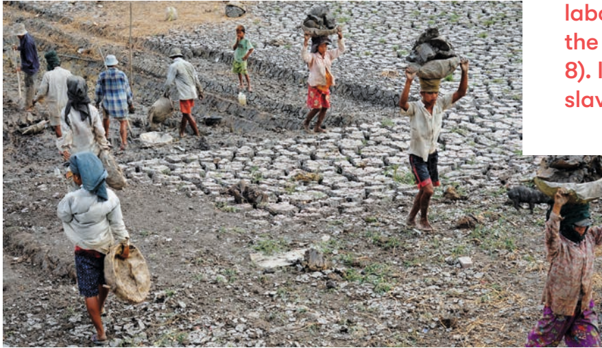
Workers on an irrigation construction site, Myanmar, 2013. © ILO, Photographer: Crozet M.
