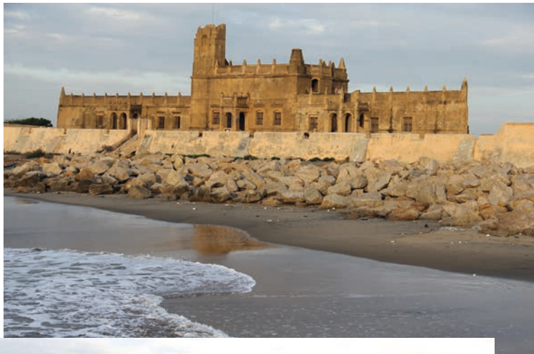
Fig. 2 (right): Danish fort at Tarangambadi constructed in 1620 by Naval Col. Ove Geddy with the permission of King Raghunath Nayakkar of Thanjavur. The fort consists of two levels. The lower level was used as godown, prison and resting area for soldiers while the upper floor was the residence of the governor and priests.
