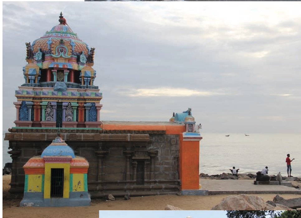
Fig. 3 (above): 14th century Siva temple on the sea coast at Tharangambadi, which continues to be worshipped by local communities.
