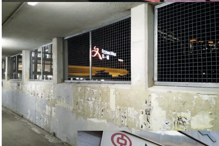
Fig. 7 (left): Newly installed grates near above Kowloon Tong metro station.
