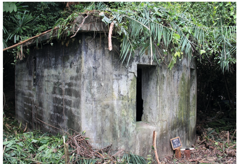
Fig. 3: One of the DEL emplacements featuring steel reinforced shuttered concrete construction to protect the searchlight equipment and crew. (Credit: Aaron Kao)
