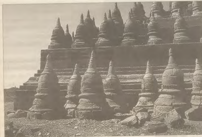
Northeast corner, exterior, after restoration. Many of the stupas have been made for the restoration (2000).
